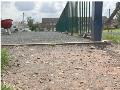
Neil to level this surface
